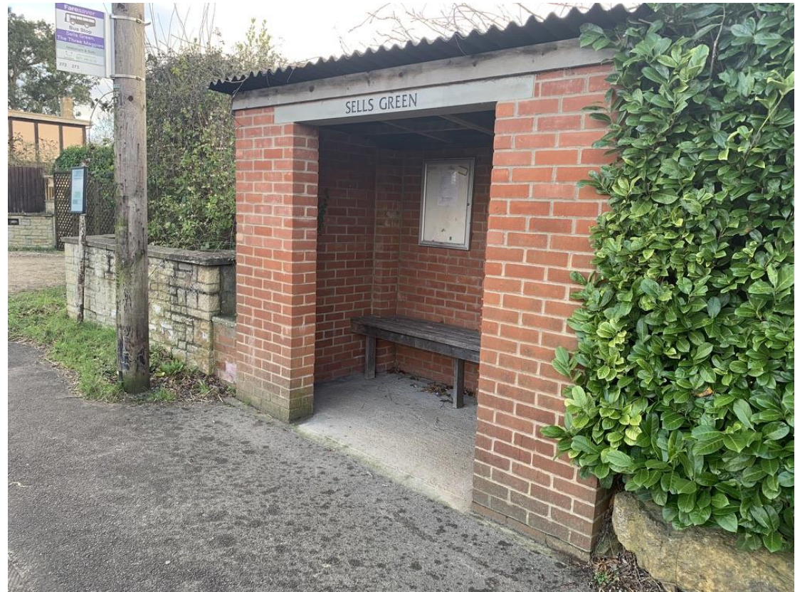
Sells Green – Westbound Bus Shelter
