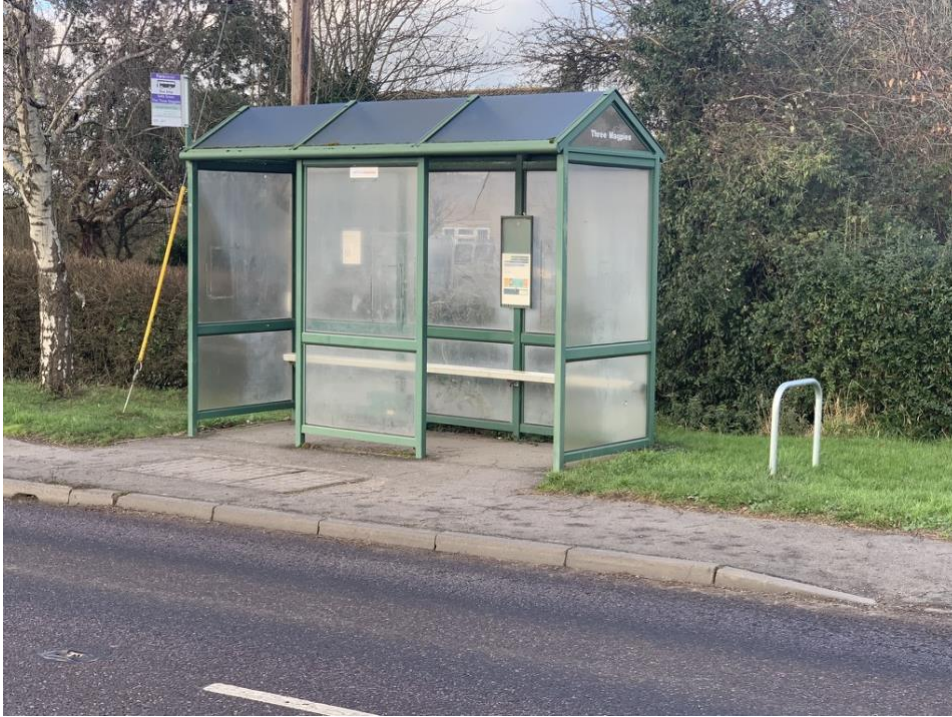
Sells Green – Eastbound Bus Shelter & Cycle Rack
