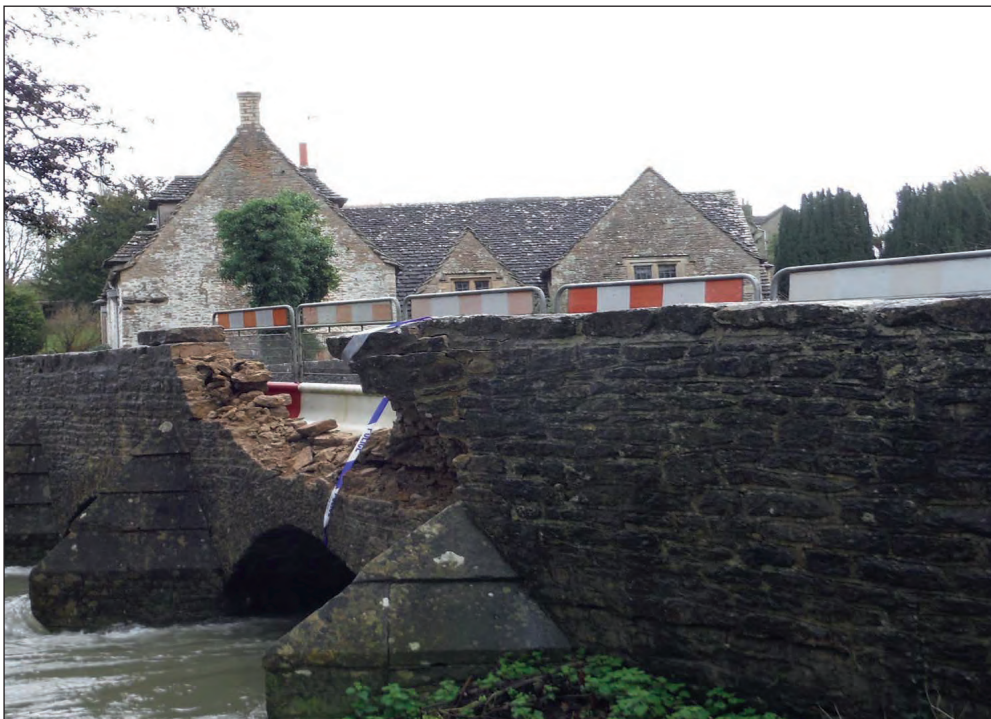
Figure 7- Damage to Baldham Bridge - Under Repair (2)
