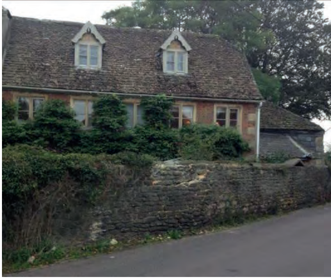
Figure 15 - Damaged wall at the 'pinch point'
