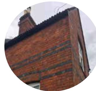
Decorative brickwork (in a Flemish Bond) with bricks used to define scale and details on the windows and chimney
