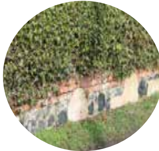
Boundary walls in Seend Cleeve feature slag and mill stones
