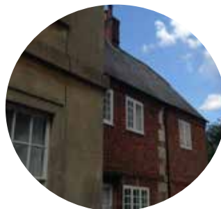
Dressed stone features in Seend especially for the larger buildings, together with the more common combination of brick and stone
