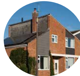
Buildings which belong to distinct architectural eras can be found in Seend - the layout and materials still sensitive to the setting
