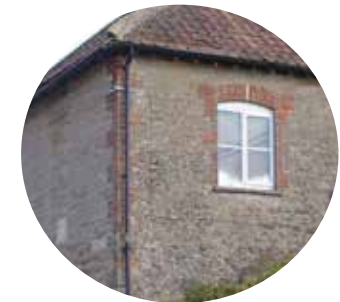
Brick quoin and architrave detailing to stone buildings
