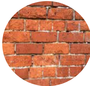
Orange brick laid in an English Garden Wall bond. A common colour and bond, particularly in Seend Cleeve
